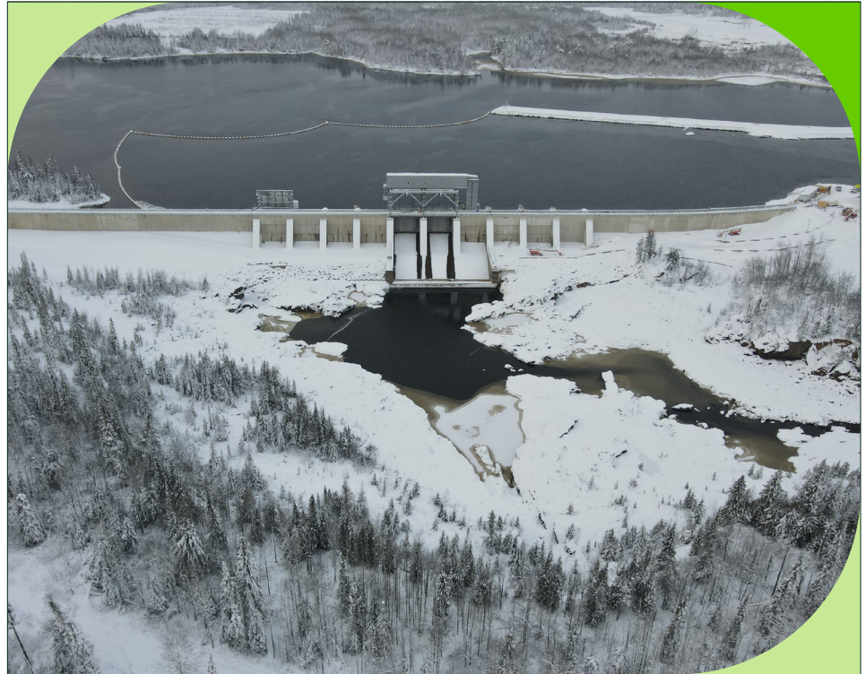
The Smoky Falls Dam Safety Project is expected to be complete in mid-2025. The project included replacing two sluice gates and permanently closing other gates that are no longer required.
